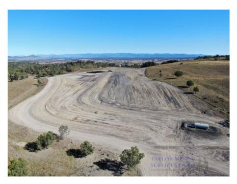
Oakleigh East showing ongoing rehabilitation and capping of a tailings dam area. Images taken from the north-east by Taylor Mining Services Pty Ltd
