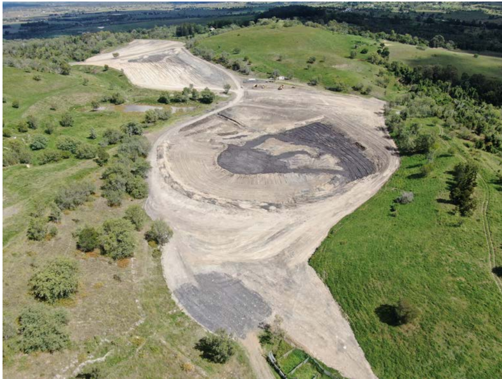
Oakleigh East showing ongoing rehabilitation and capping of a tailings dam area. Images taken from the north-east by Taylor Mining Services Pty Ltd
