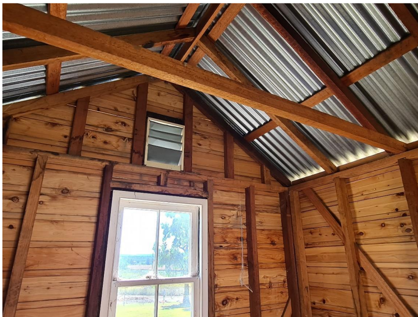
Reconstructed garden shed internal view of cladding and framing
