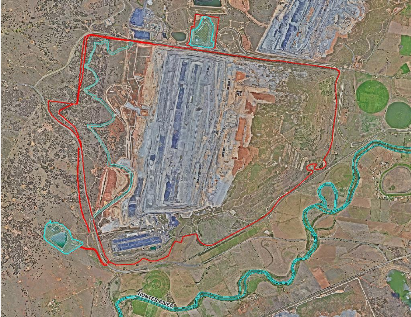
FIGURE 8: Site Clean Water Diversion Dam and Levee and Hunter River
