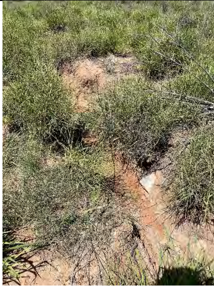
Photo 4 – Example of Gully erosion
