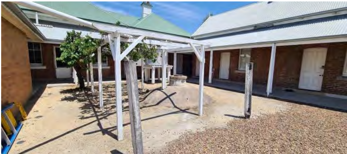
Main homestead, northern aspect
