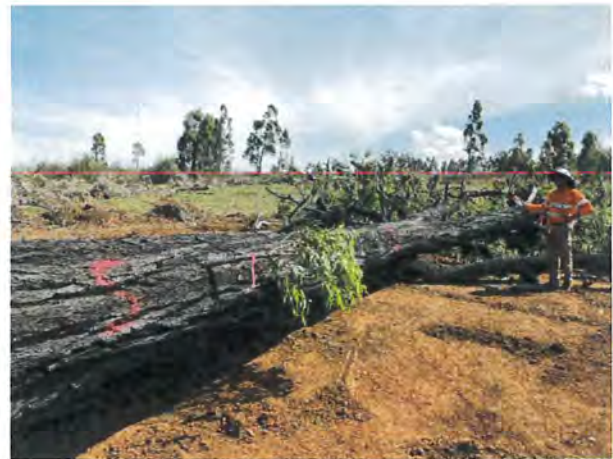
Photo 3.5 An example of salvageable material identified during Stage 2 tree clearing
