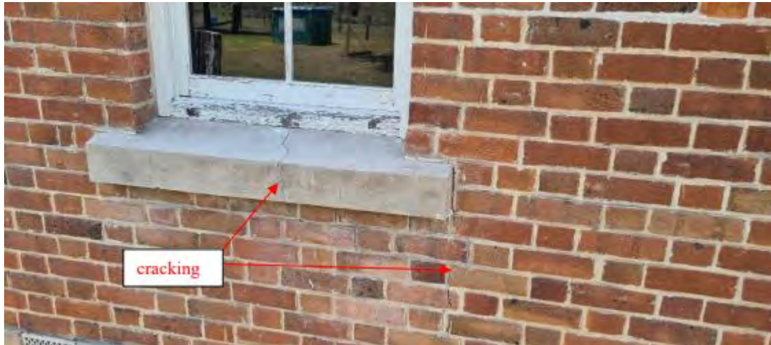
Example of brick and mortar repairs needed
