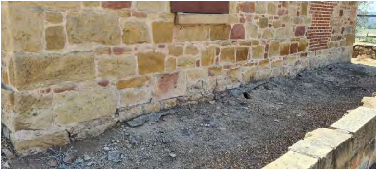
External view of exposed verandah area
