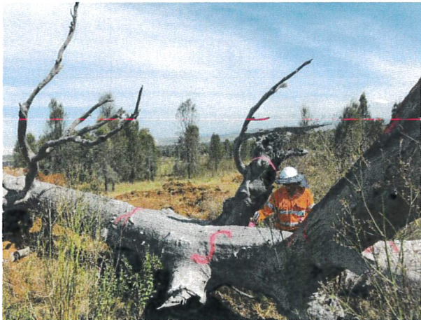
Photo 3.4 An example of salvageable material identified during Stage 2 tree clearing
