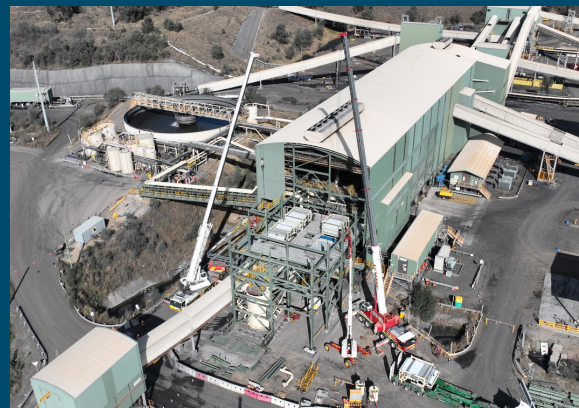
CHPP Growth Construction
