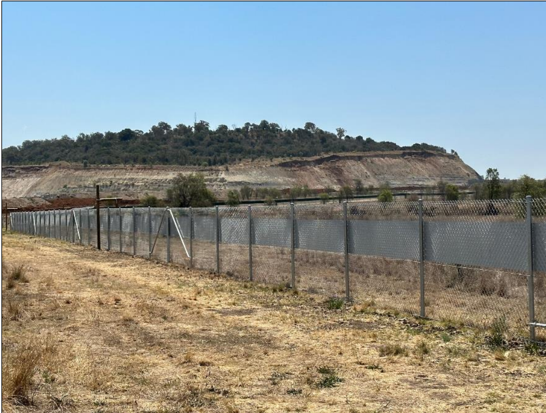
Photo 2 Koala exclusion fencing near future haul road crossing
