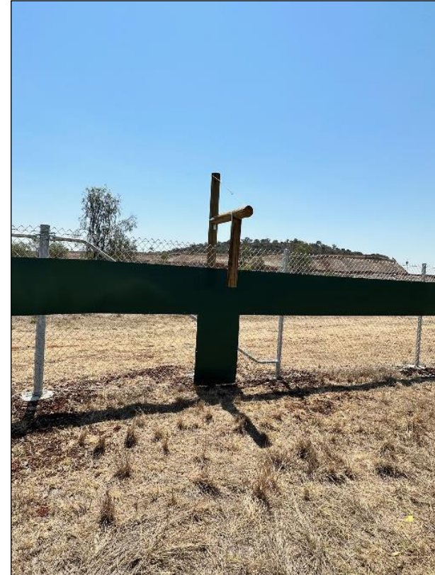
Photo 3 Koala exclusion fencing showing timber exit pole
