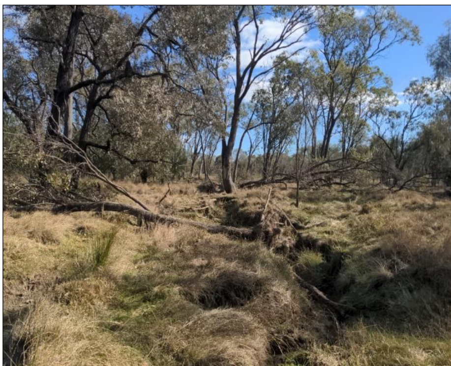
Lagoon Creek erosion causing tree fall near LC09
