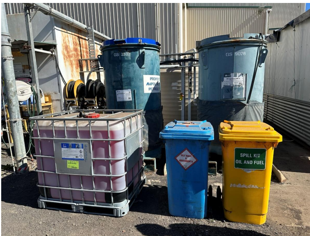
Photo 12 Radiator coolant stored outside bunded area. Labelled spill kit and waste bins in place.
