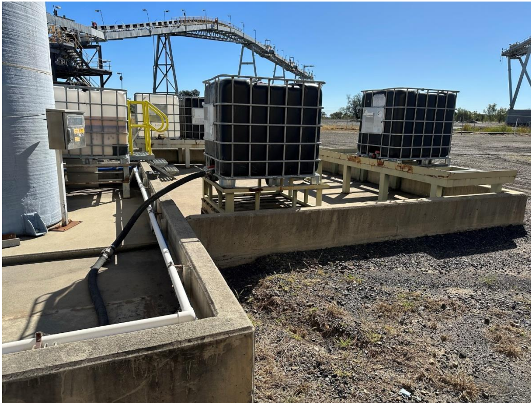
Photo 12 Radiator coolant stored outside bunded area. Labelled spill kit and waste bins in place.
