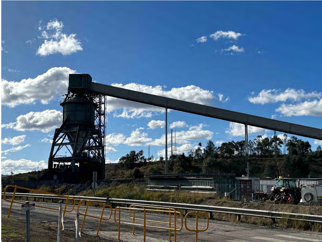
Plate 5 - CHPP Reject Bin
