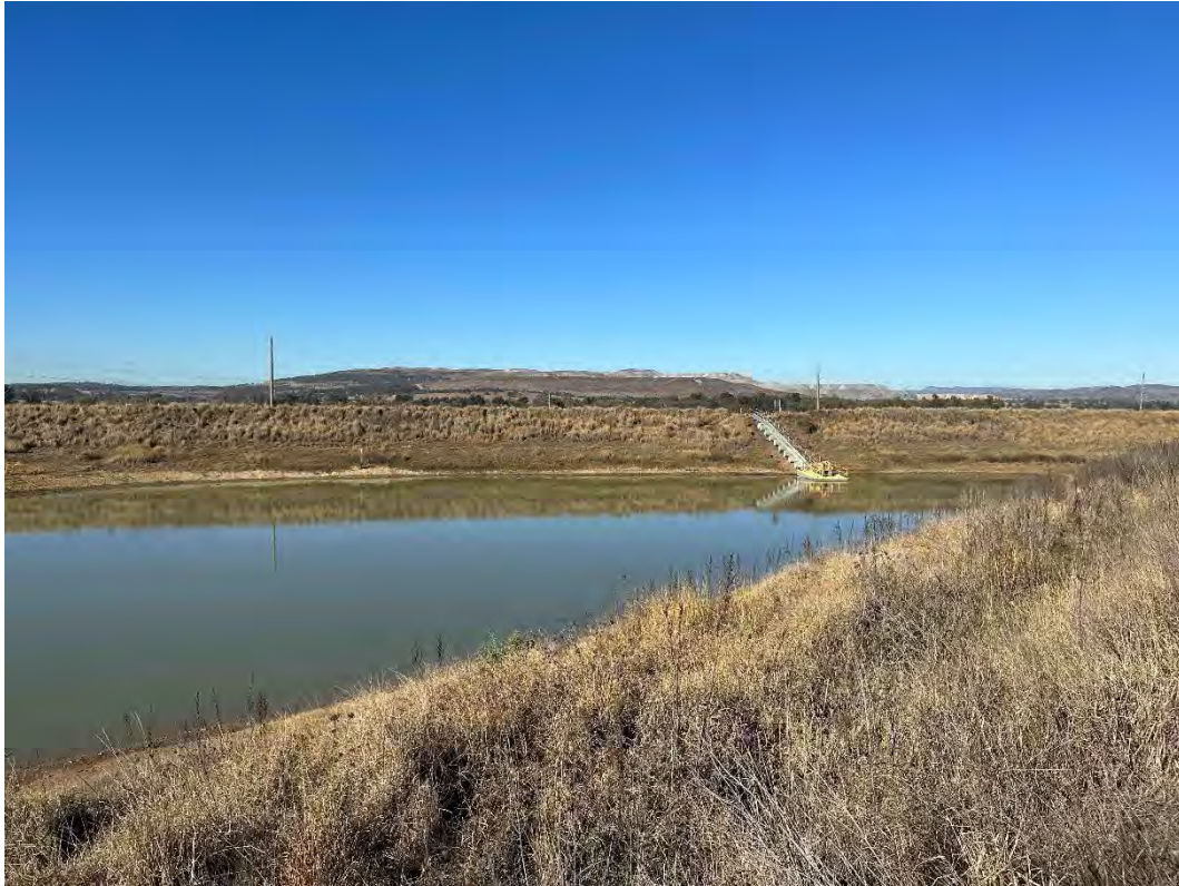
Plate 11 - End Wall Dam
