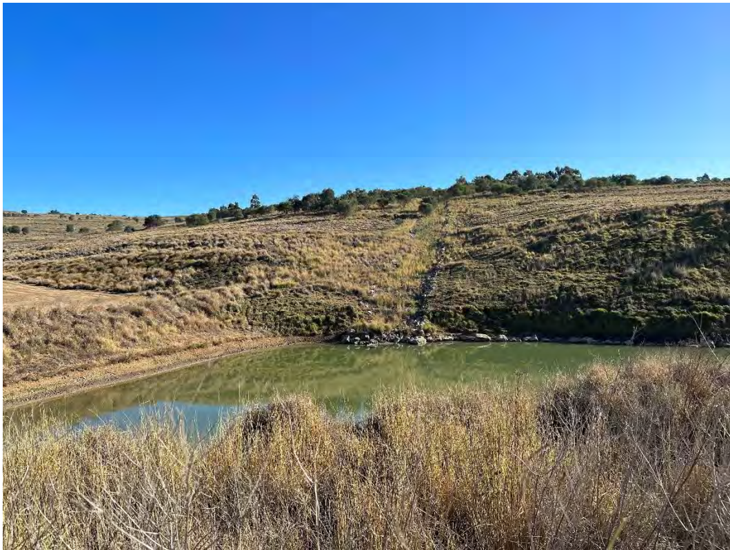
Plate 10 - End Wall Dam
