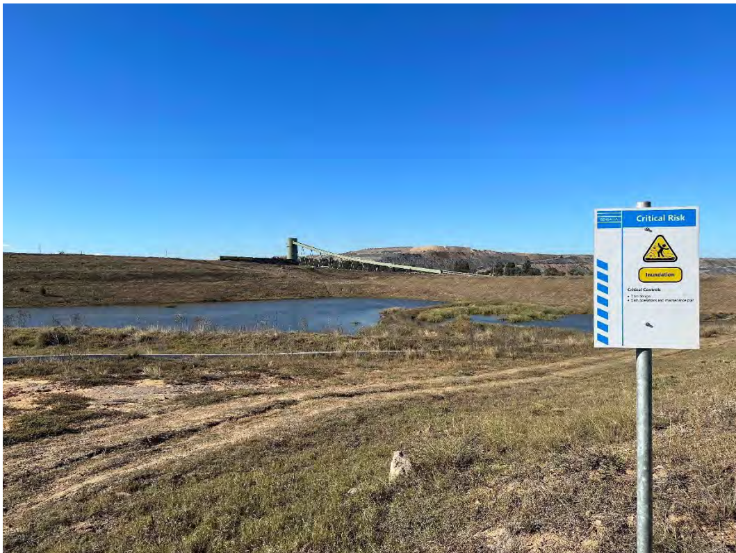
Plate 12 - End Wall Dam
