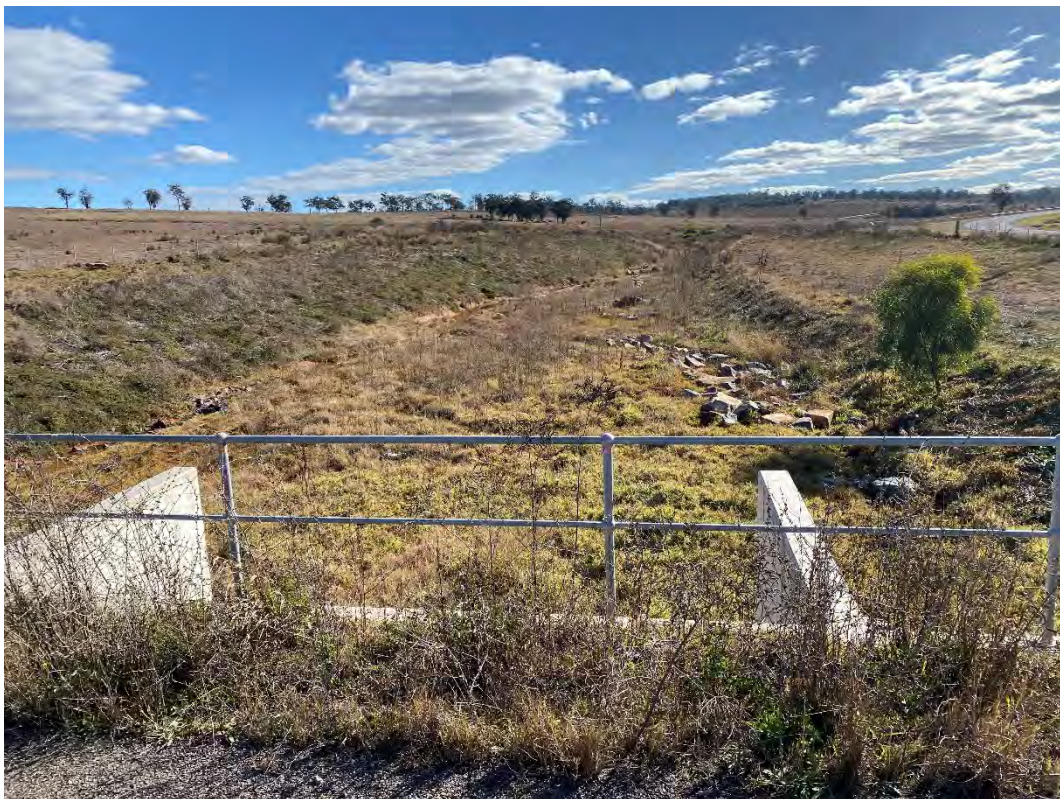
Plate 28 - Dam Drainage System
