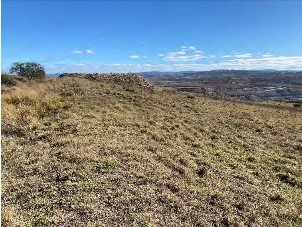
Plate 33 - Lack of Rehabilitation on Northern Face
