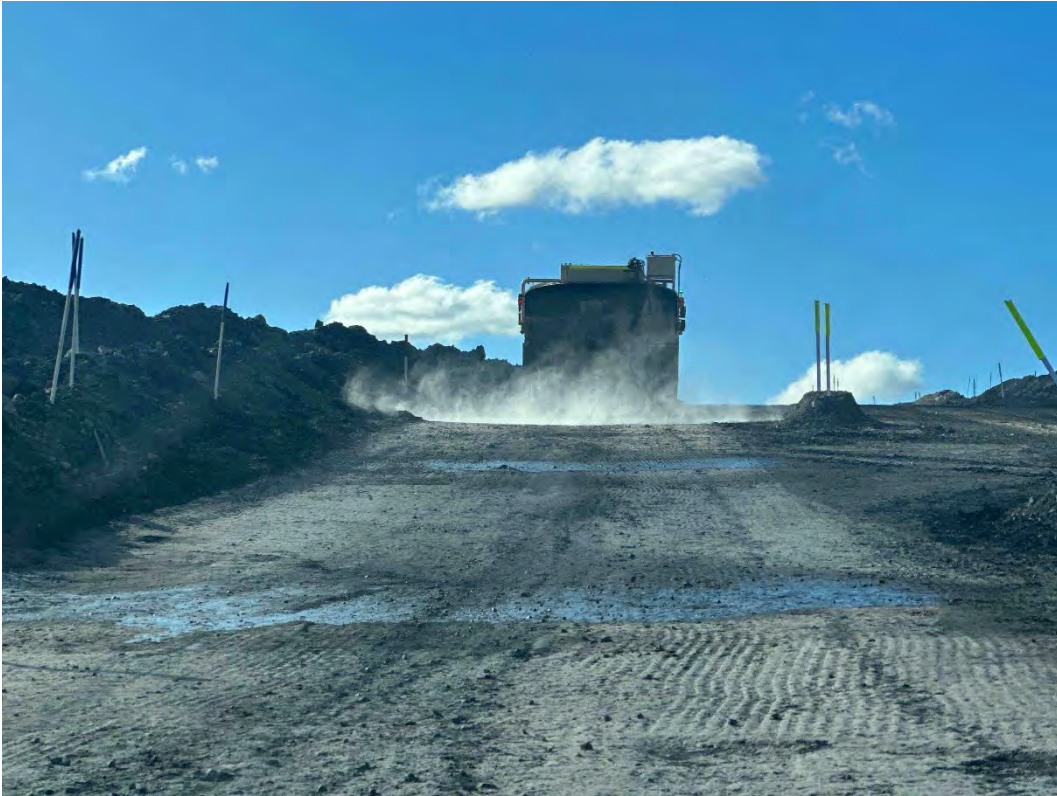
Plate 7 - Water Cart on Haul Road
