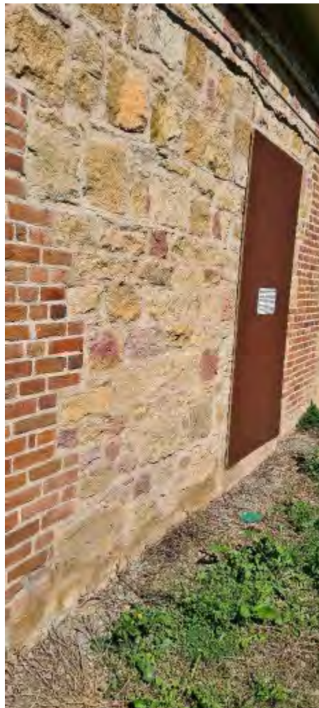
'Overdene', western elevation
