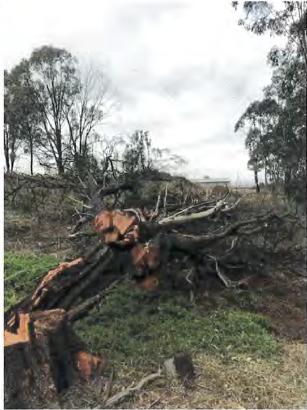
Photo 3.6 Stage 2 – clearing – post felling
