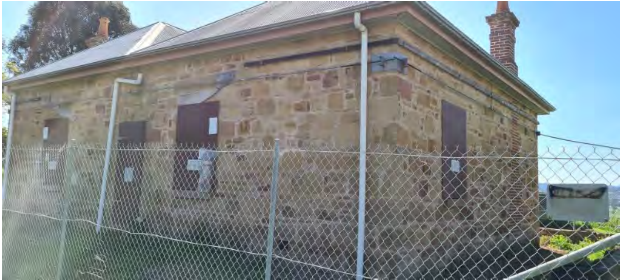
'Overdene', typical southern elevation
