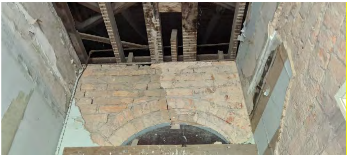
'Overdene', Internal Passage
