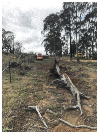
Photo 3.12 Stage 2 tree clearing operations associated with the electricity easement
