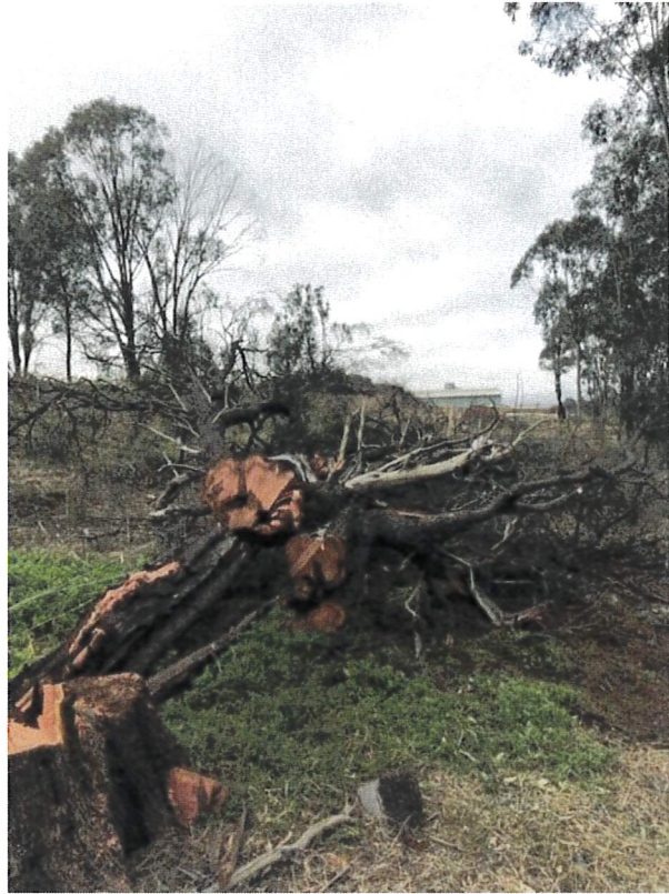
Photo 3.6 Stage 2 – clearing – post felling
