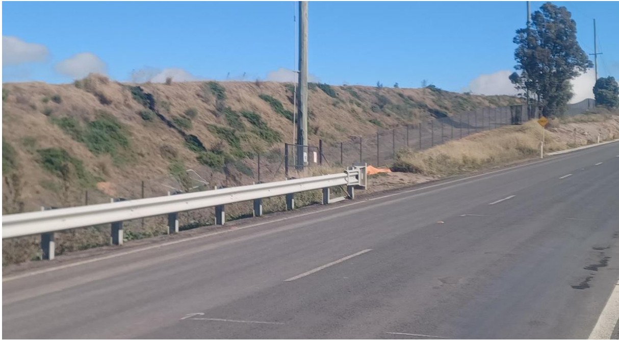
Figure 8 Photo of a visual bund located adjacent to Wybong Road on the mine site looking generally West to Bengalla
