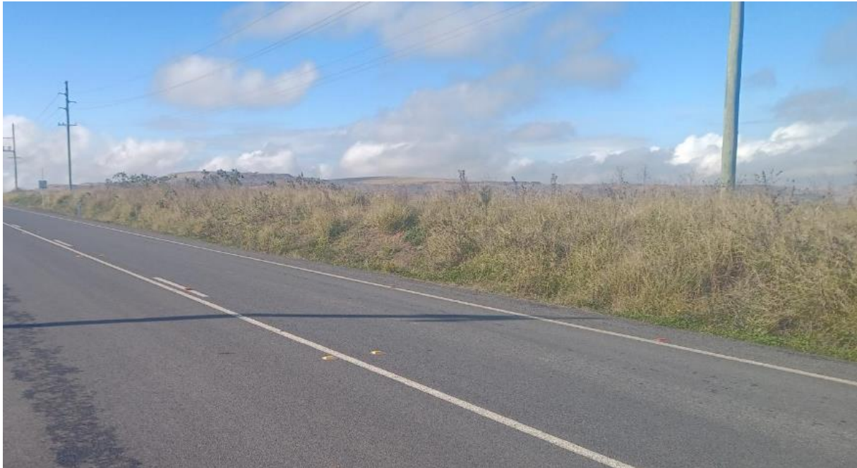
Figure 6 Photo of Wybong Road cutting looking generally East to Bengalla
