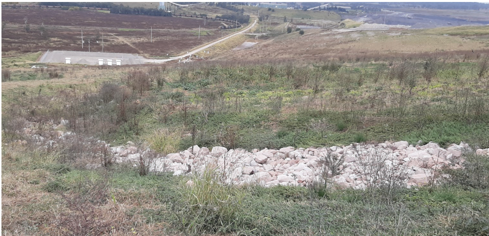
Bengalla landform showing installed natural drainage line
