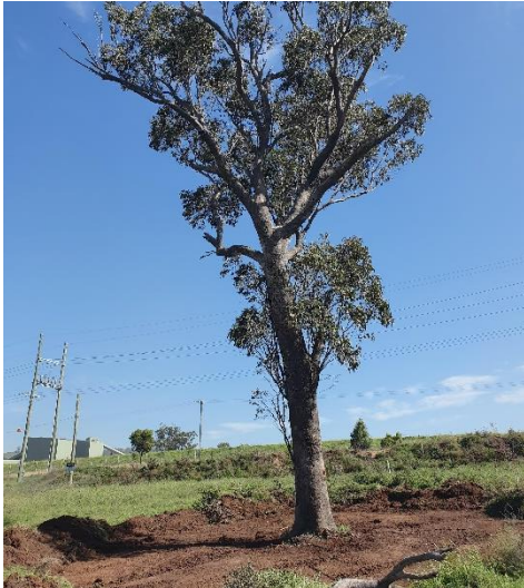
Photo 3.1 Stage 2 – clearing – GDP 2101
