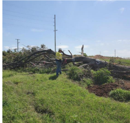
Photo 3.2 Stage 2 – clearing – post felling
