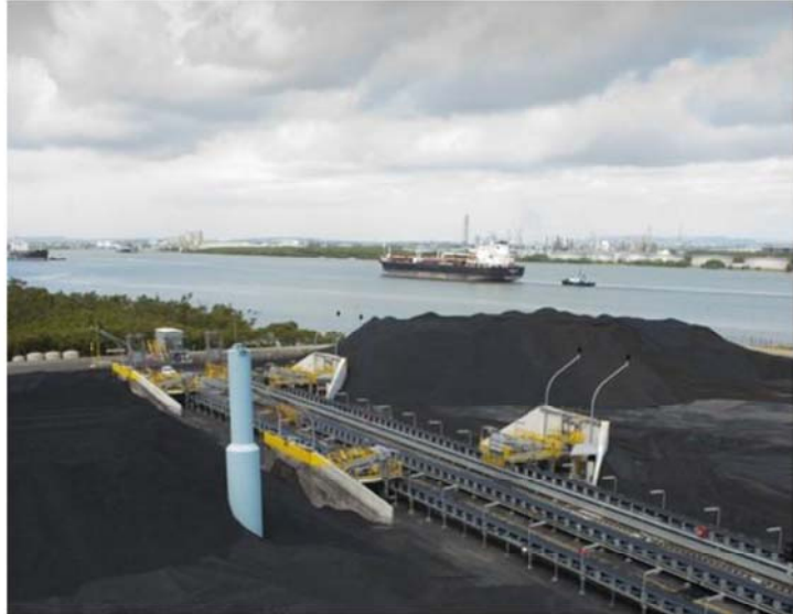
Figure 14: QBH operations at the Port of Brisbane
