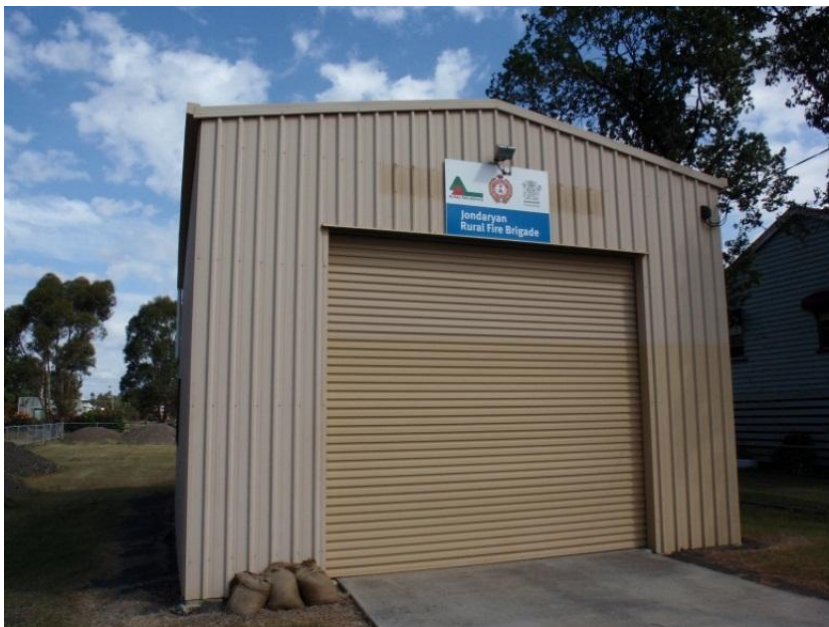
Photograph 16-4 Jondaryan Rural Fire Brigade Shed
