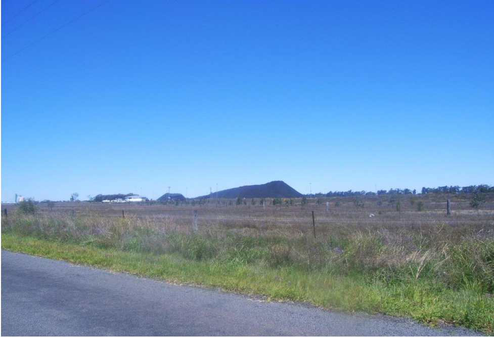
Photograph 15-5 Existing Jondaryan Rail Loadout Facility
