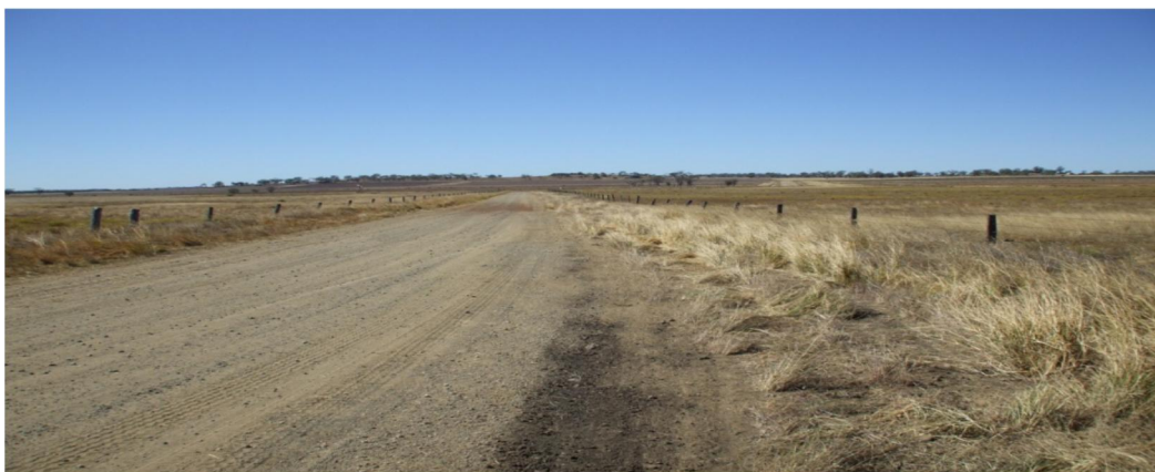
Photograph 13-1 Childs Road at the rail crossing (view to the east)
