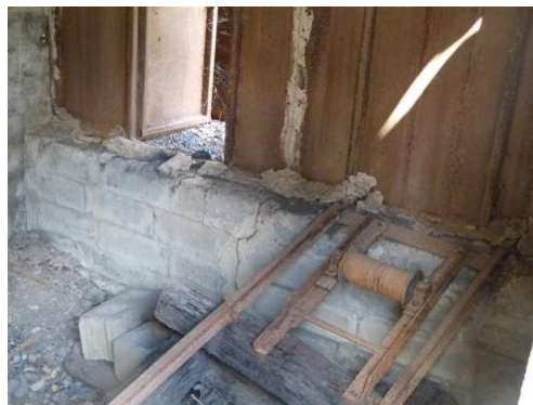
Photo 122 – Railway Tracks inside Structure
