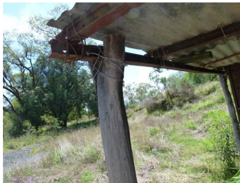
Photo 66 – Awning Rail Track Beam to Post Fixing
