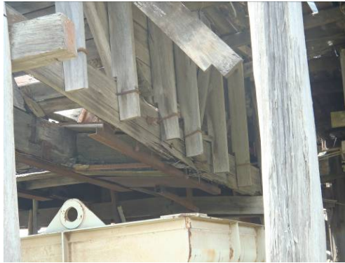
Photo 40 – Broken Hopper Joist and Broken Internal Bearer
