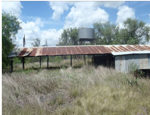
Photo 22 – North Elevation (Rear) – Pit Head Entry
