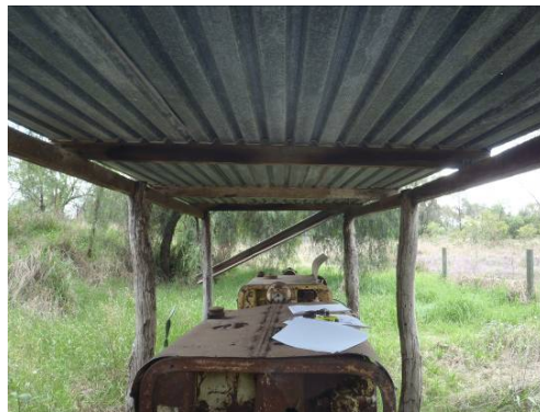
Photo 4 – Typical Roof Framing
