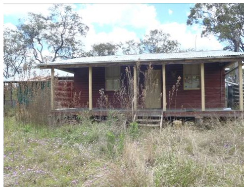
Photo 6 – Front Elevation of Manager's Office
