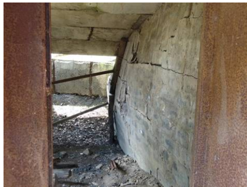
Photo 121 – Eastern Internal Wall Braced
