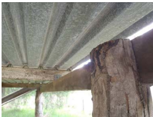
Photo 5 – Typical Fixing Detail
