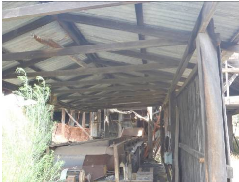
Photo 24 – Interior of Picking Belt Shed
