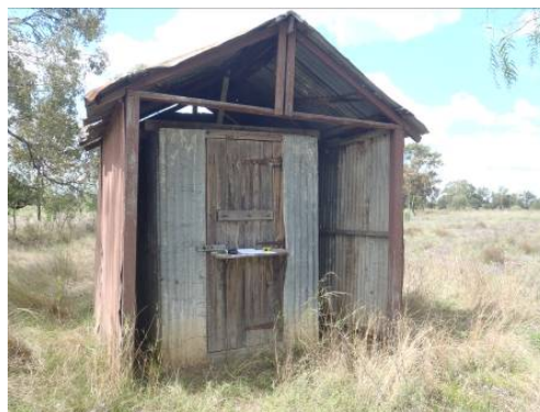
Photo 17 – Front Elevation of Explosive Shed
