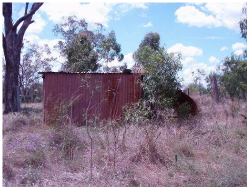
Photo 51 – Rear Elevation of Shed
