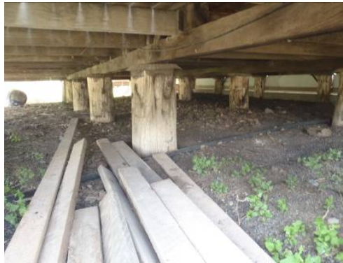
Photo 10 – Subfloor Framing and Fixings
