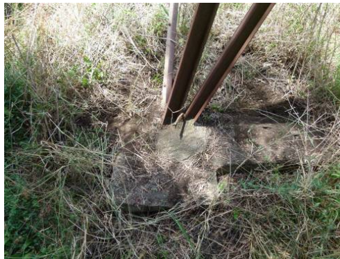
Photo 83 – Concrete Foundation of Water Tank 500 X 500mm
