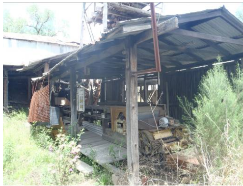
Photo 25 – View of Picking Belt Shed
