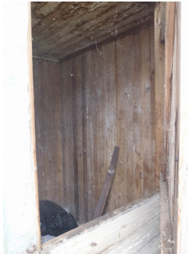
Photo 18 – Internal View within Explosive Shed
