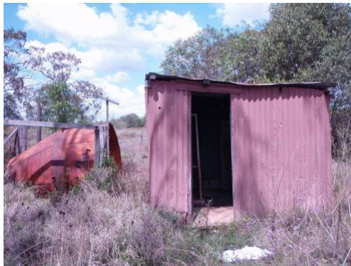
Photo 50 – Elevation of Shed and Fan Cowl
