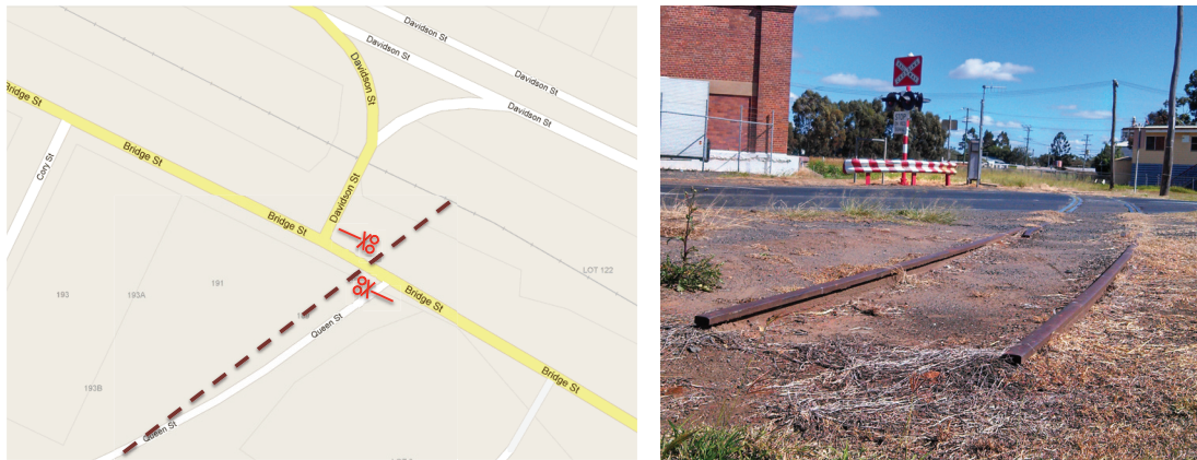
Figure 9: Unused level crossing on Bridge Street
