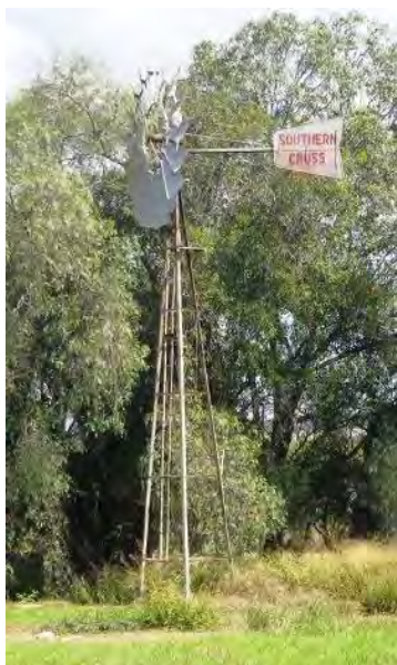
Photo 3 - The windmill located near Tom Doherty Park will be maintained (17 George Street).
