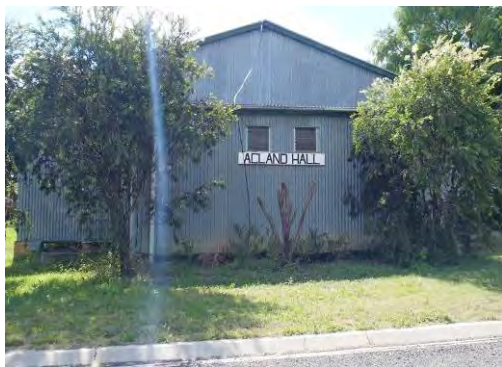
Photo 2 - Acland Hall, which will be maintained and utilised by NHG under the current Acland Management Strategy (2014).
