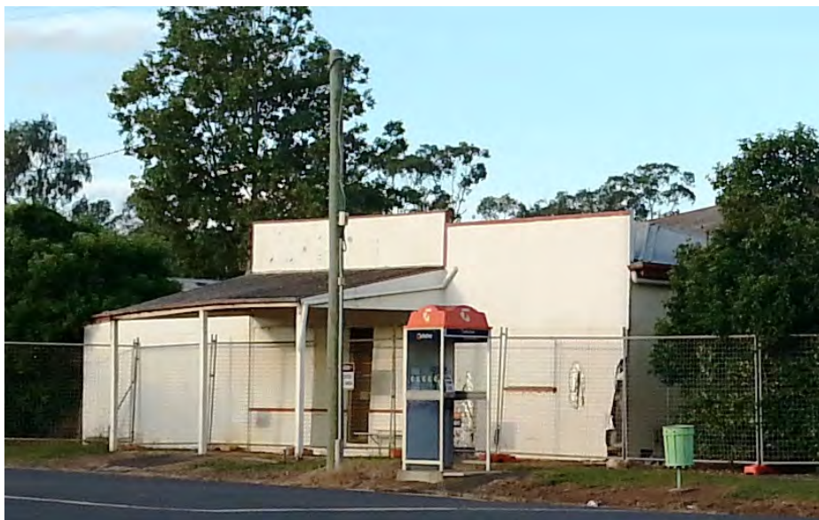
Photo 5 - Derelict former Acland store prior to demolition.
