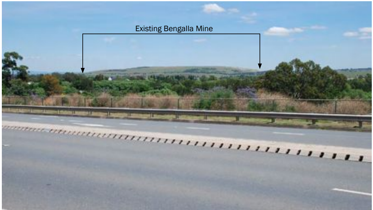
Figure 5.2 | View of main OEA from East The existing OEA is broad flat topped landform providing screening to mine activity.
